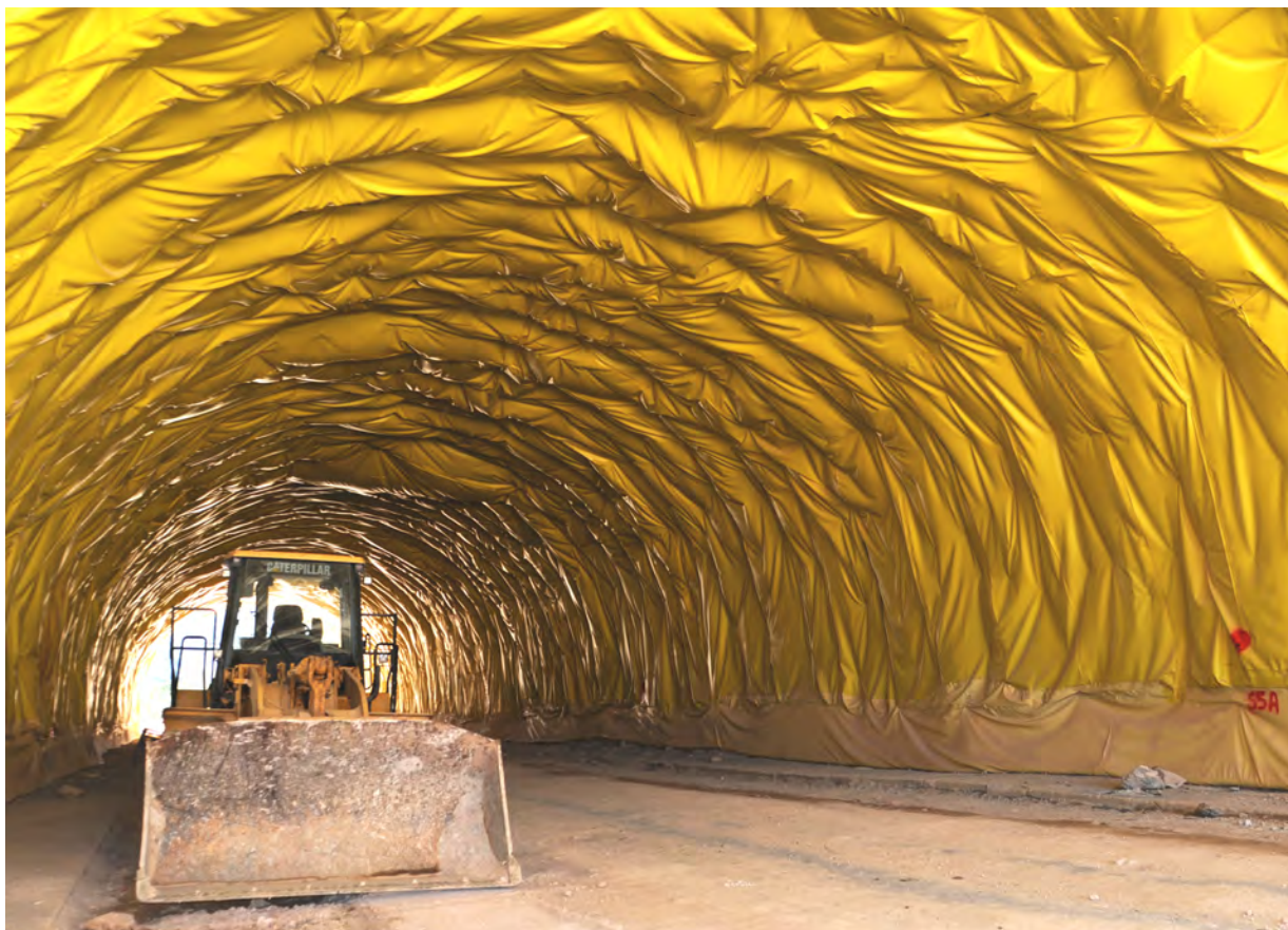
Túnel Magueyal, Carretera Durango - Mazatlán
